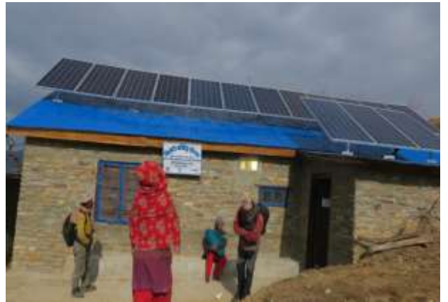
Birthing Centre at Bhadgau, Jumla
